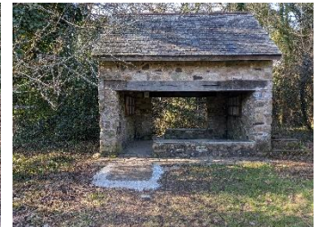
Access ramp to the Linhay
