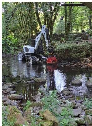
Balfour Beatty have started their work under the railway viaduct to install scour protection on the bridge piers. The nature of their work involves delivering rocks and concrete sections to the site. They do not anticipate noise disturbance, but you will notice construction traffic around Vicarage Road bridge where the road crosses the railway.
